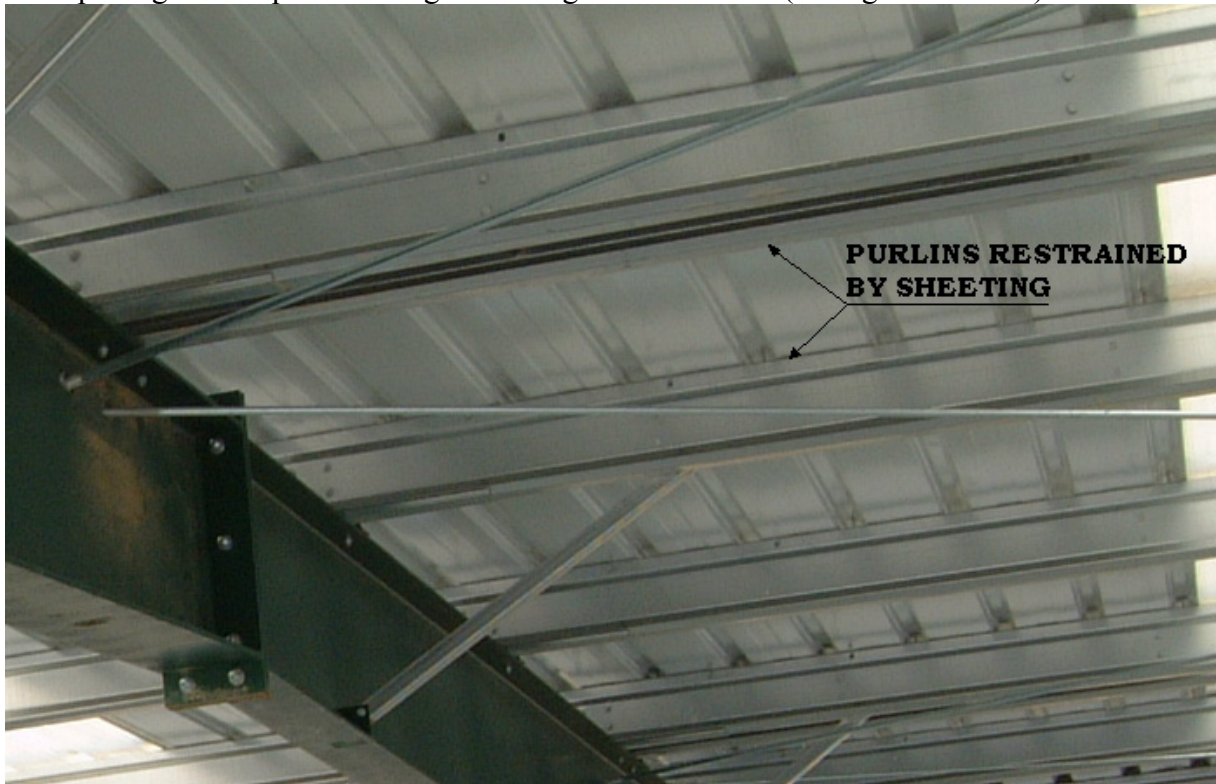
Fig. 1 – Cold-formed purlins restrained by sheeting
